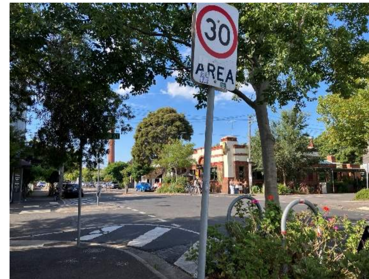
Gold Street / Hotham Street: linemarking used to visually narrow intersection
