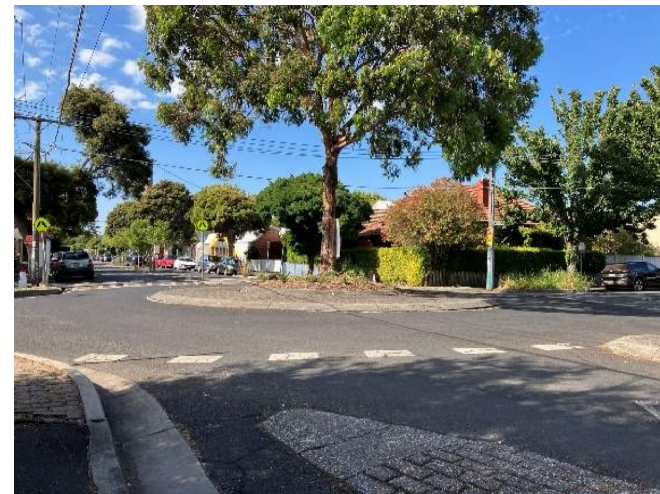
Gold Street / Keele Street: kerb islands and a raised crossing on the northern leg
