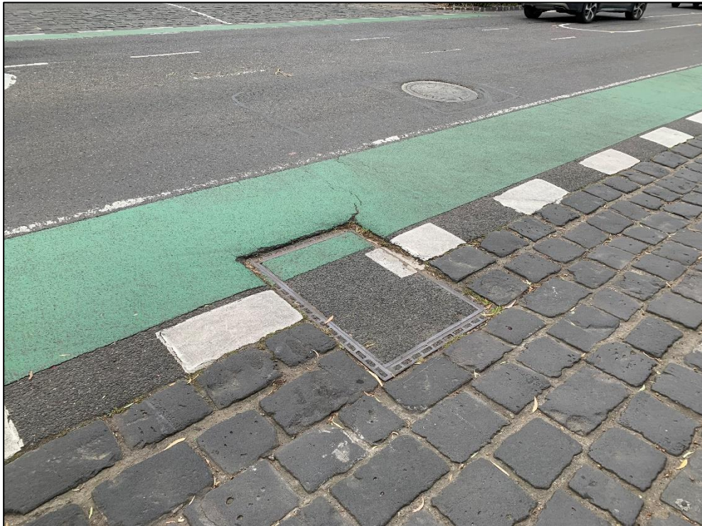
Photo 2: Depressed drain cover within the bicycle lane, at the Wellington Street and Sackville Street intersection
