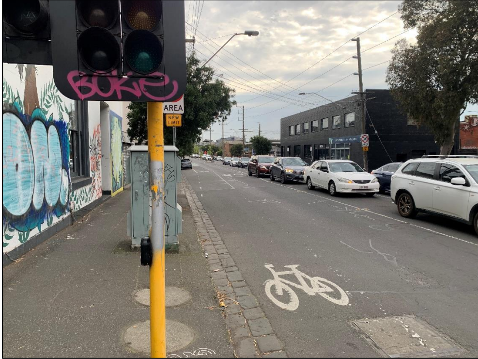
Photo 2: Depressed drain cover within the bicycle lane, at the Wellington Street and Sackville Street intersection
